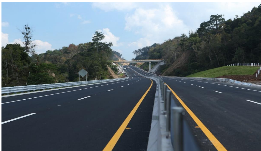
COPEXA highway (Mexico)
